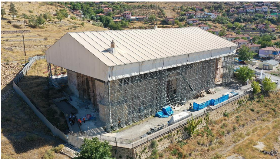
Image 3: Restoration Work at Great Mosque and Hospital of Divrigi
